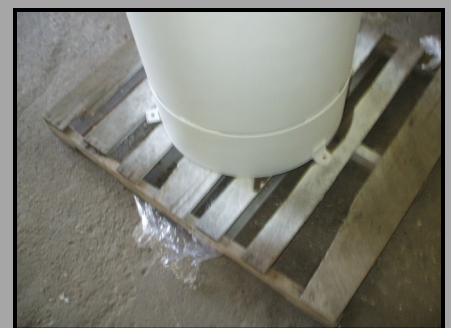
Feet are welded on tank
