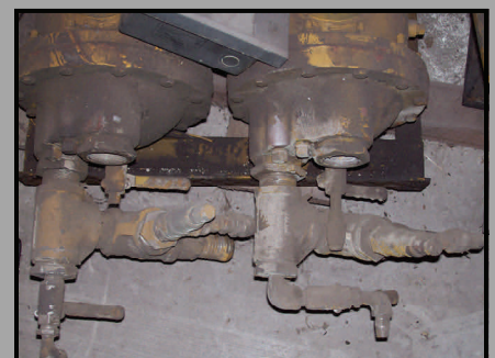
Heat exchangers equipped with air actuated water flow control valves.
