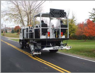
Simultaneous center & edgeline striping
